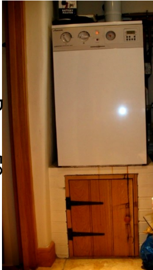
Boiler raised up
